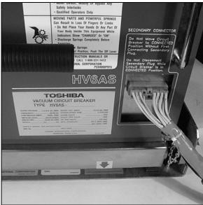
Fig. 23 Breaker at DISCONNECTED Position
